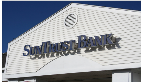
examples of internally illuminated channel letter signs; SUNTRUST letters appear dark blue during the day and white at night
